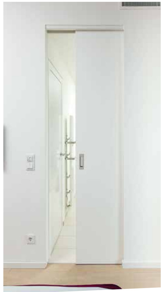
Porta deslizante na parede, vista exterior / Sliding pocket door, outside view
